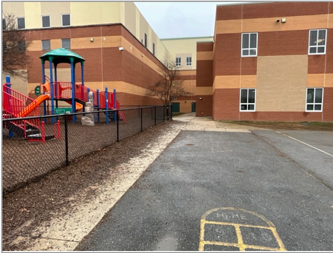
ACCESSIBLE ROUTE TO PLAYGROUND
