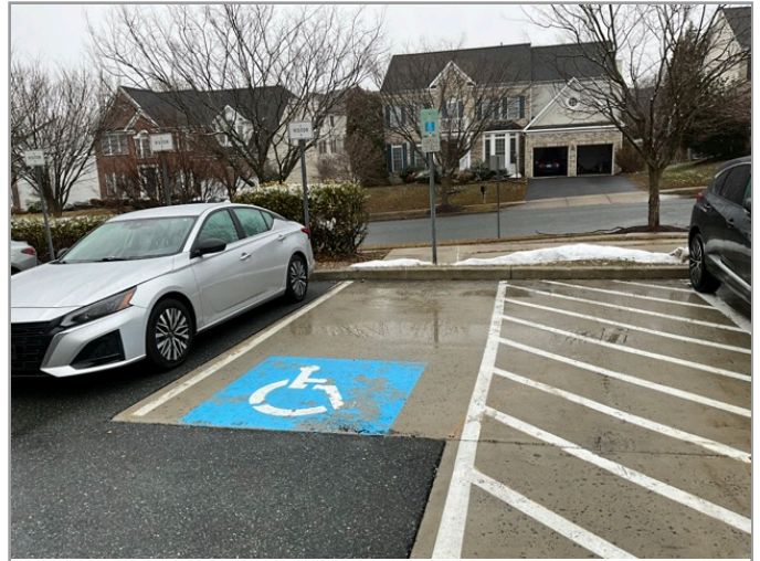
OVERVIEW OF ACCESSIBLE PARKING AREA
