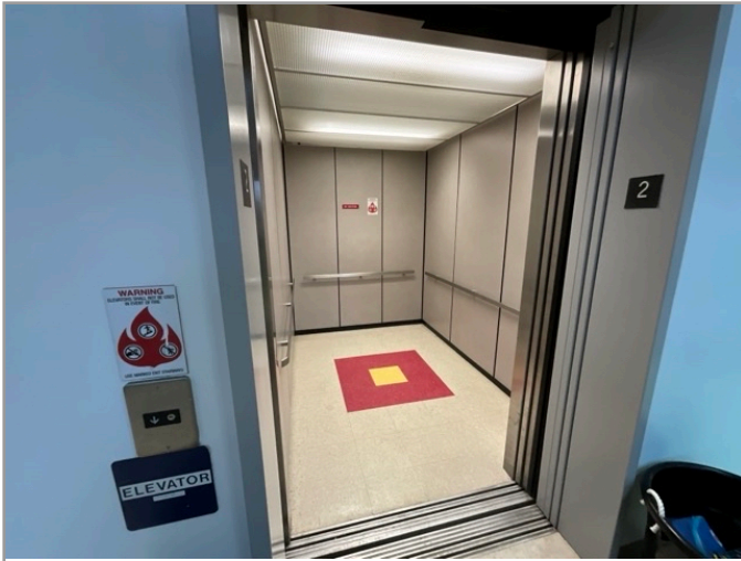
LOBBY LOOKING AT CABS (WITH DOORS OPEN)
