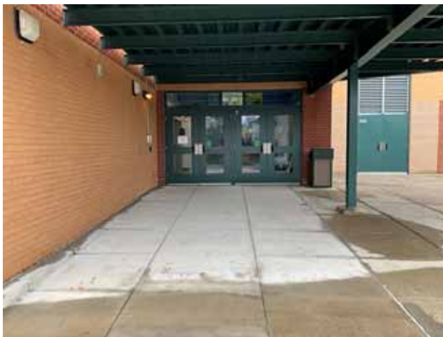
5 - WALKWAY TO ENTRANCE
