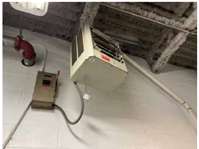
18 - TYPICAL UNIT HEATER
